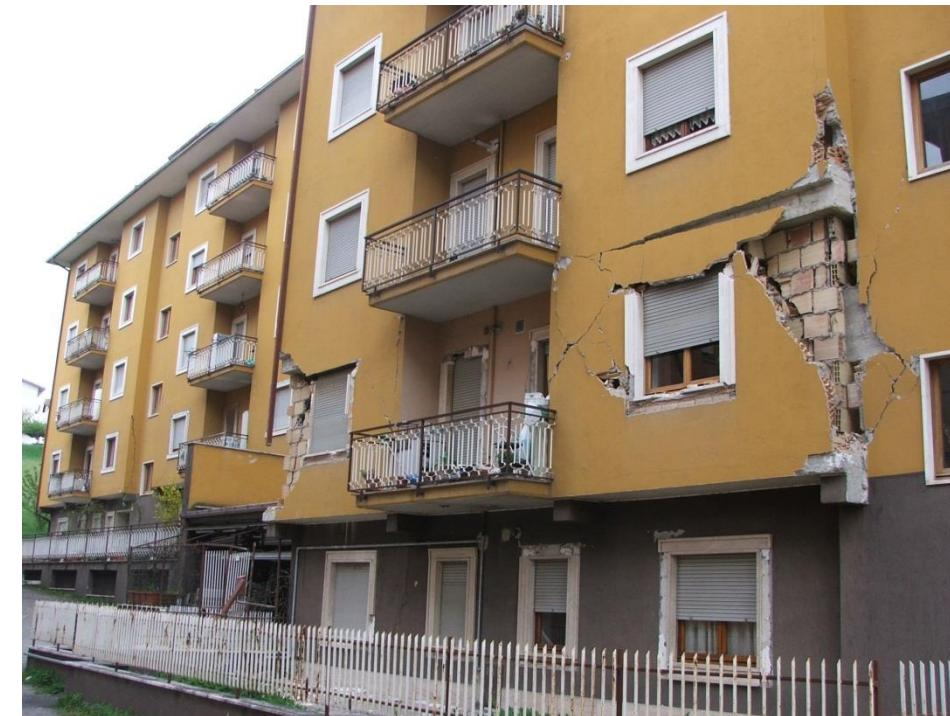
L'Aquila 2009 – Residential buildings with damage to bow-windows under high vertical seismic actions
