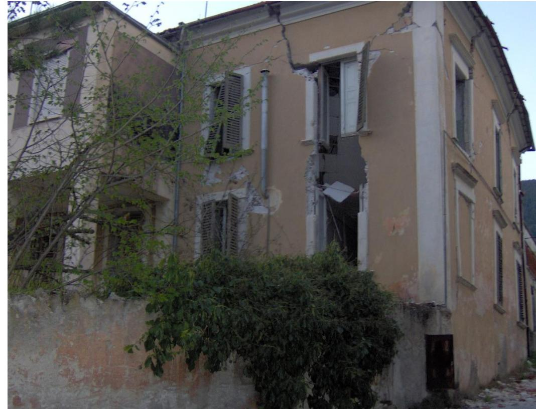
L'Aquila 2009 – Residential buildings with damage due to high vertical seismic actions
