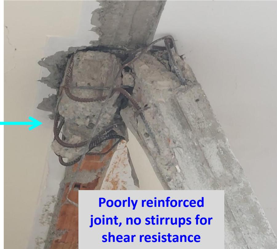
**Poorly reinforced joint, no stirrups for shear resistance**
