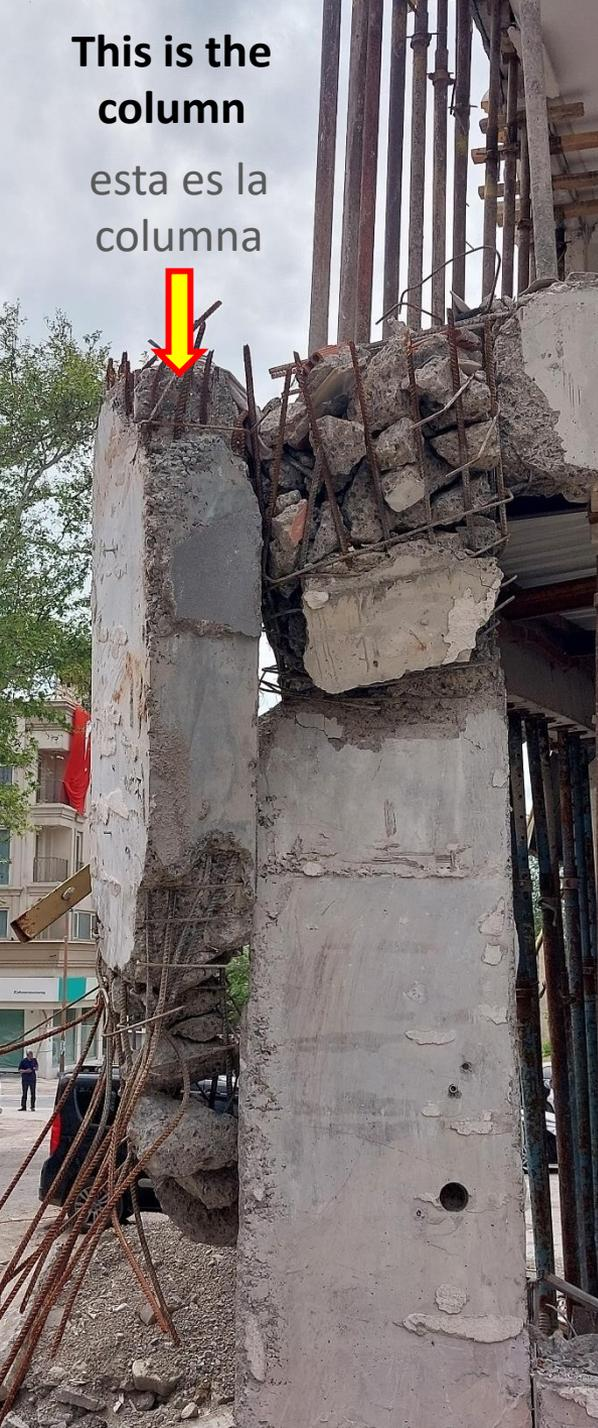
**Longitudinal reinforcement is discontinued at the joint**
